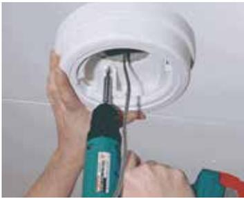
Step 1: Secure Housing to Mounting Surface
