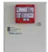
This Series 1948 12V 0.5A PSU module is mounted lower down in this version of the compact cabinet to allow the Centaur Cube ASE to be mounted at the top. A cutout is included in the door for the ASE (no blanking plate is fitted). There is also space for 1 x 12V 7Ah battery.
